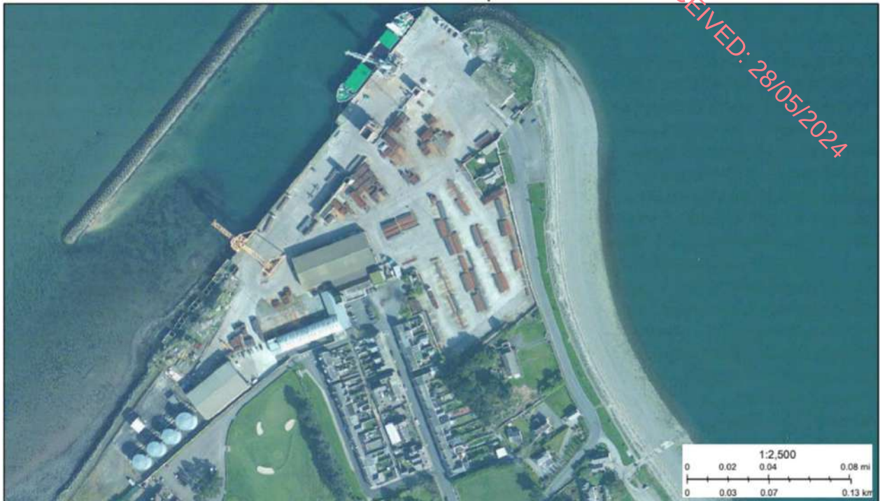
Figure 2-10 OSi Aerial image from 2013 (OSi, 2023)
